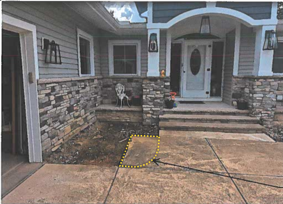
PROPOSED CONCRETE REMOVAL
