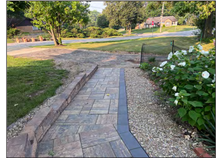
EXISTING WHEELCHAIR ACCESS
