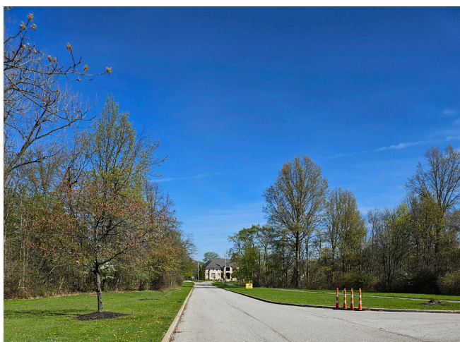
Existing Perimeter - North Drive
