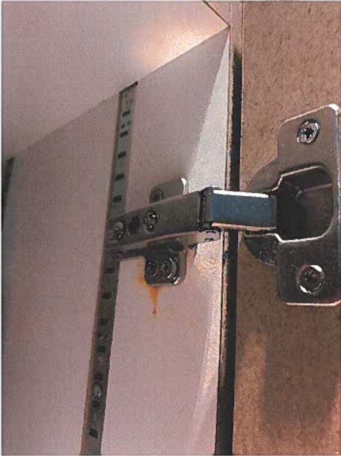
Glue holding cabinet together
